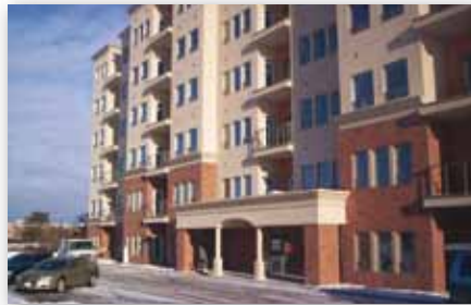
Nottinghill Gate Oakville Ontario, Canada
